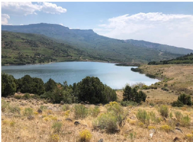
Palisade Drinking Water, Cabin Reservoir
