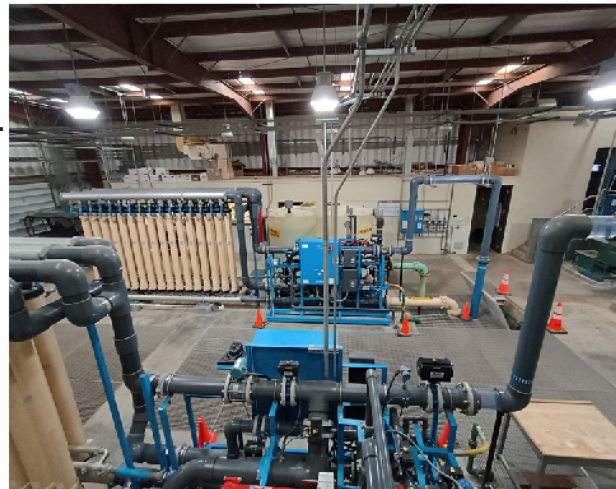
Palisade Water Treatment Plant
