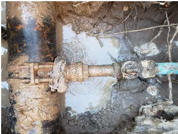
Leaking at the threads under rag.
