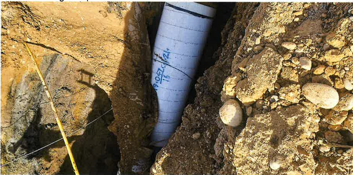
Ute water pipe is white
