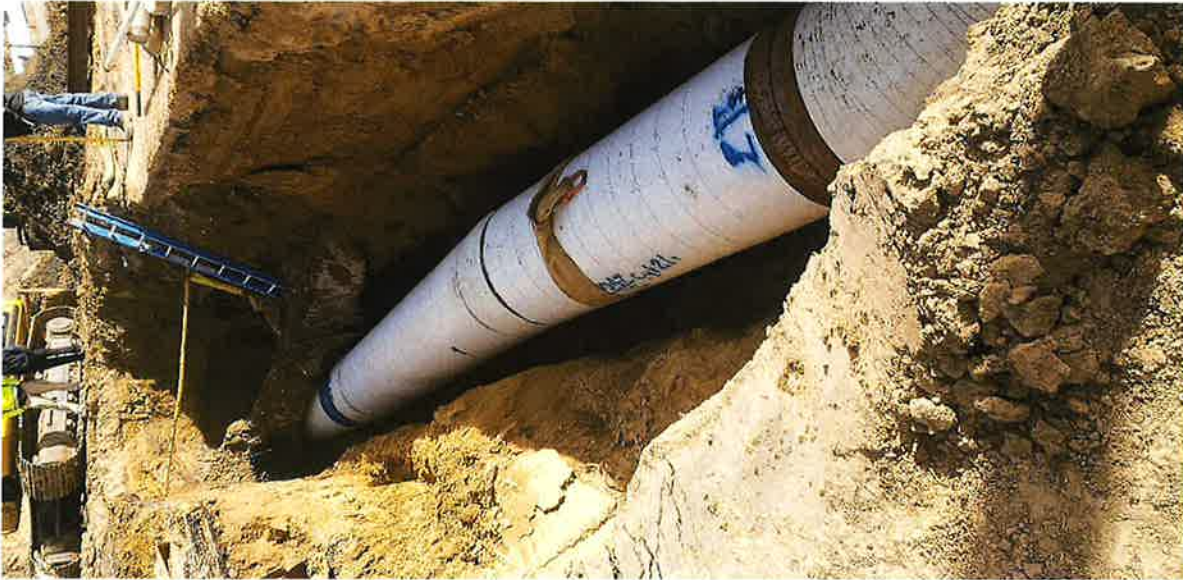
(Ute Water line in trench before the joints were welded.)
