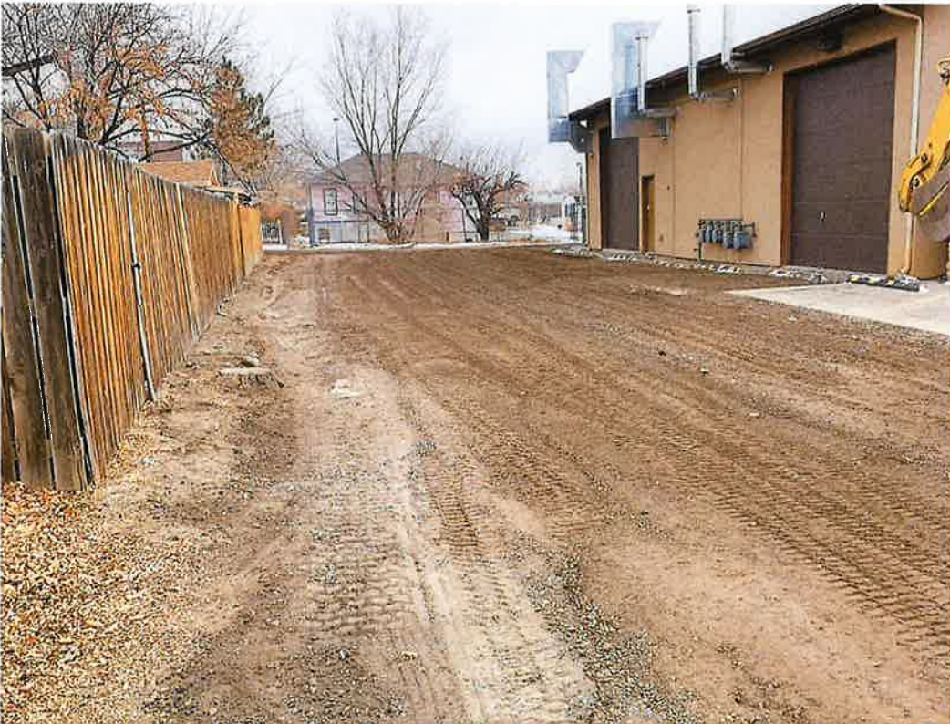
(After with a smooth grade away from the building and slight grade to Peach Street.)
