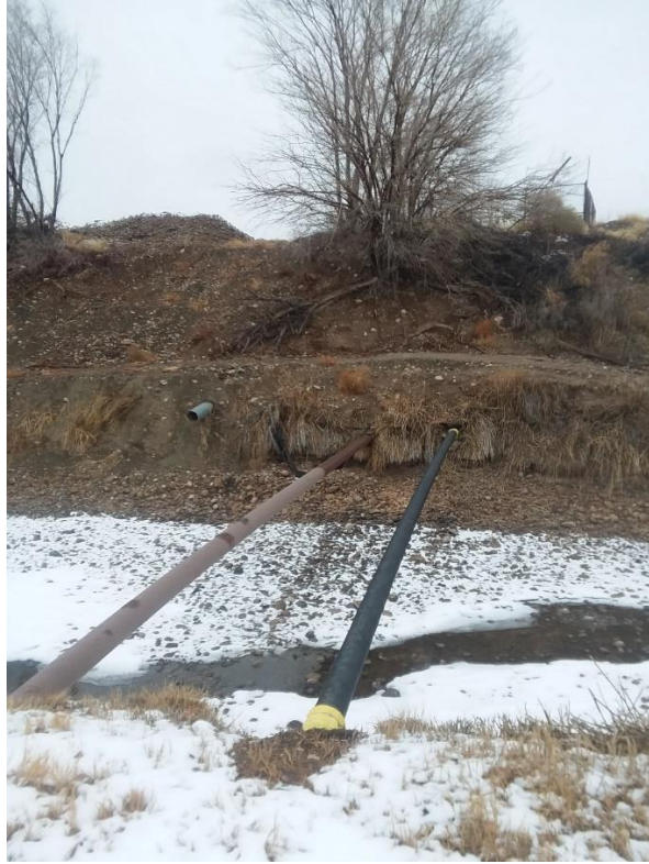
Photo #3: Riverbend Park along GVIC canal. Two lines crossing canal, sewer (west) and gas (east).
