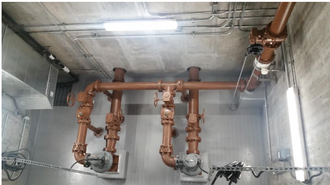
Figure 5 Pumps Inside Dry Pit
