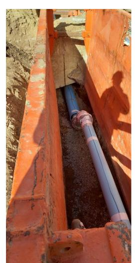
Canal crossing under canal 13 feet deep. You can see the tracer wire taped to the pipe for future locating the service. Hard to see a larger PVC sleeve for the main water line to pass through. This is the standard procedure for water lines to cross other critical infrastructure such as this canal. This shows the complexity we faced with our Elberta water leak last fall. Only a clean
