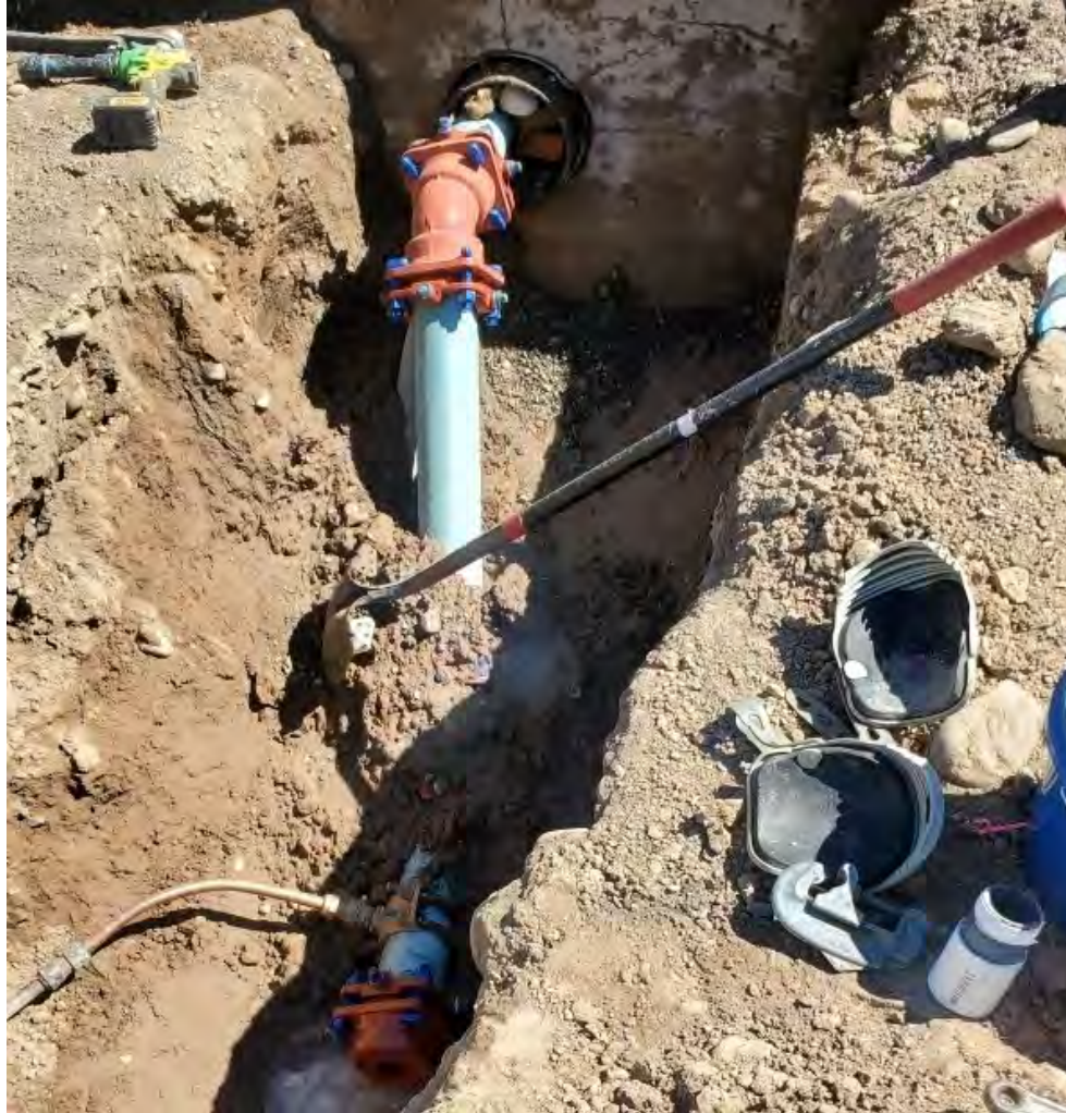
Figure 1: 4-inch Certa-lock main with mega-leg restraint joints.
